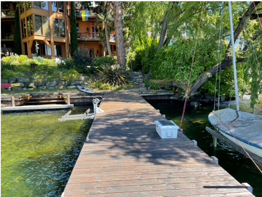
Photo 2 - Existing dock looking landward.
